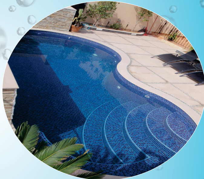
Swimming Pool Filtration
